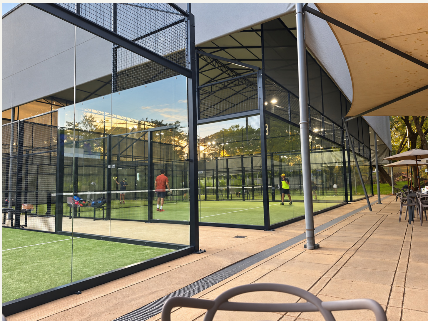
Court enclosure, roof cover and terrace viewed together.
